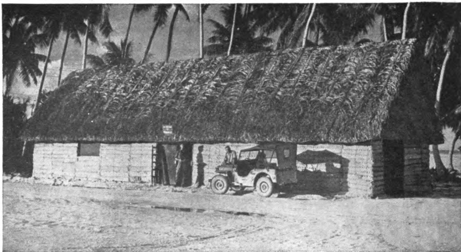
Figure 148. Warehouse constructed of local material.
